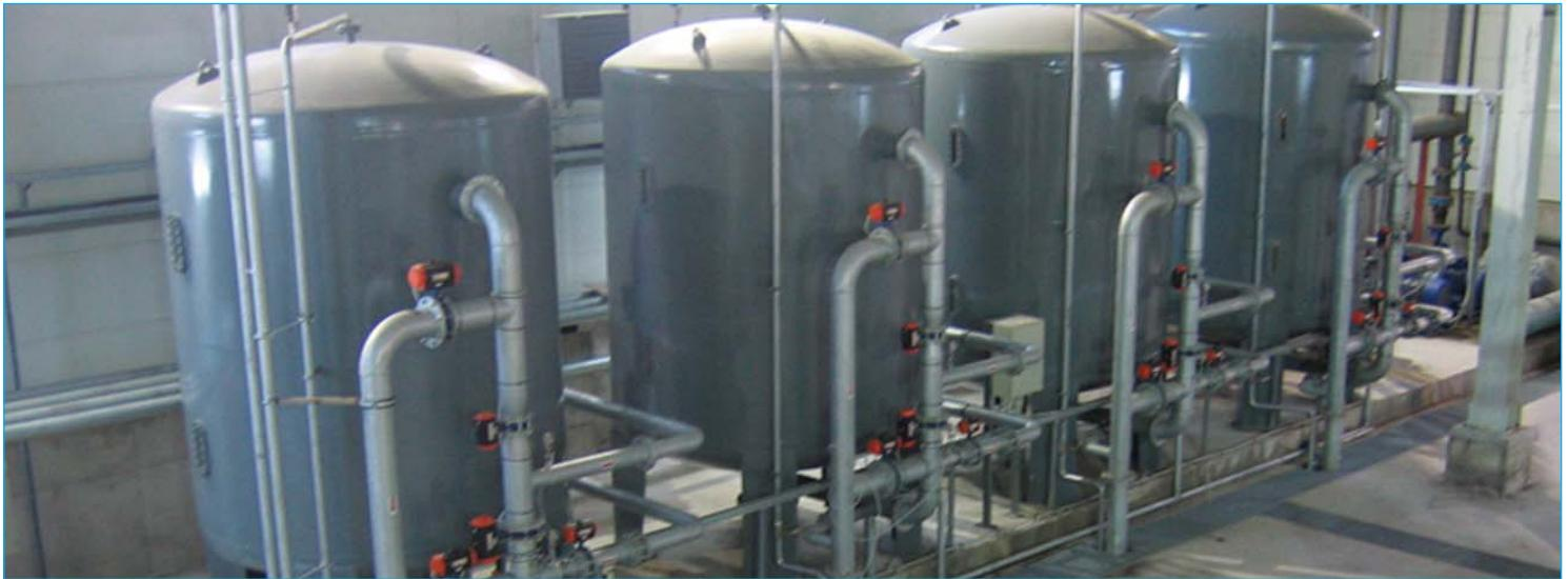
Aquasis Multi Media Filters are used for purpose of removing suspended solid, cloudiness and other particles. System is consisting of settling different degree of gravel sizes with more than one layer inside the body.
